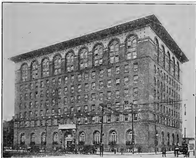
ASSOCIATION BUILDING, CLEVELAND, OHIO.
